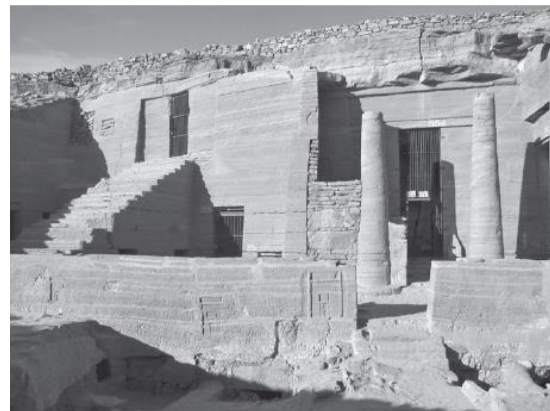
(Fig. 4- b) Staircase that provided the only means of access to (tomb 35)
